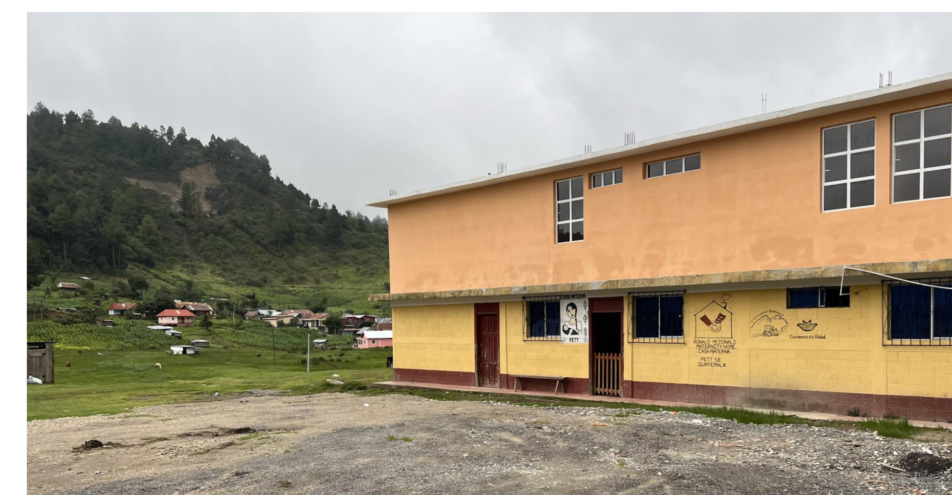
Figure 2: Casa Materna building located in Pett, Santa Eulalia
